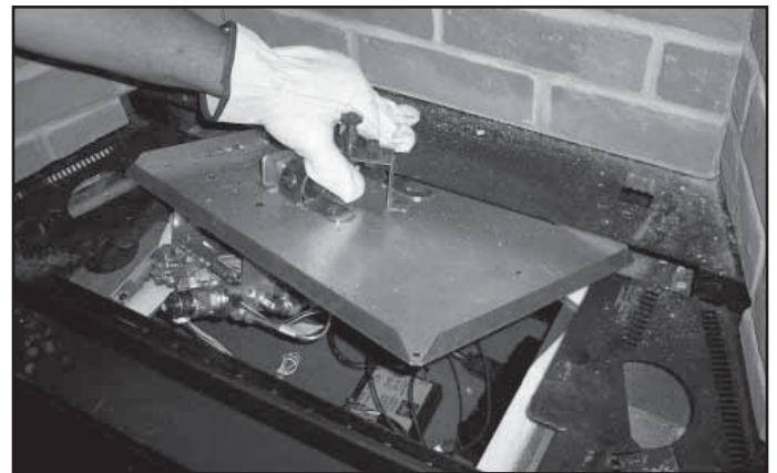
Figure 3.6 Lift Up & Remove Valve Assembly
